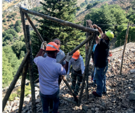
Fig. 35. Placement of a gate
