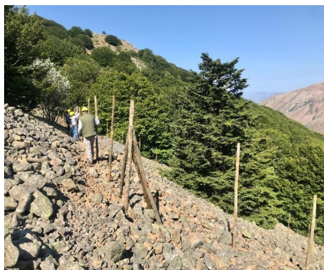
Fig. 3 – Installation of the fence
