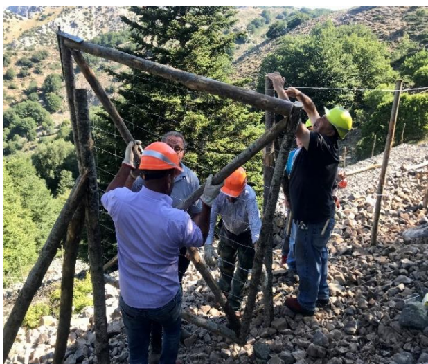
Fig. 2 – Installation of the gate
